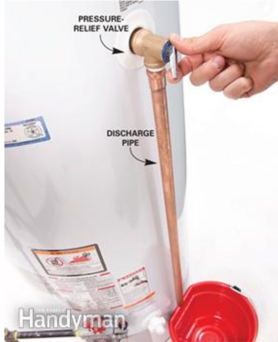
Photo 1: Check the pressure-relief valve
