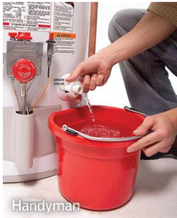
Photo 1: Check the pressure-relief valve
